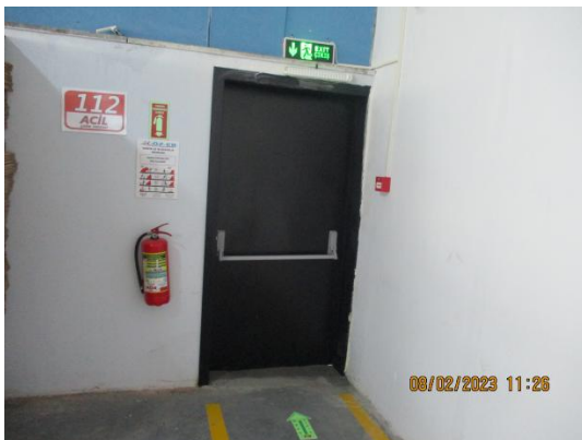
Emergency Exit Door.JPG
